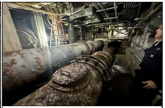
November 18 th – Electrical Work – Main PS Basement
