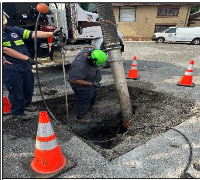
July 31 st – Excavator Crew – Little Falls
